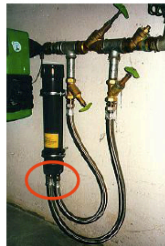
The activator installed underneath the water tap with connections facing downwards .
